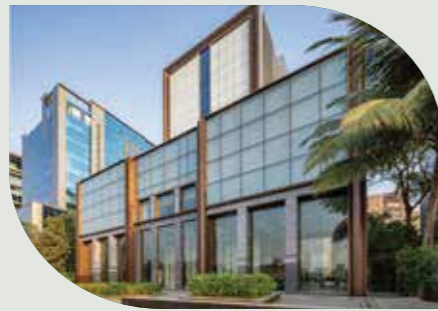
The Square Avenue 61 (BKC), Mumbai Region
