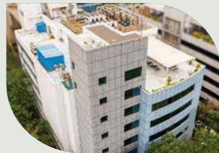
Pune IT Building (Raheja Woods), Pune
