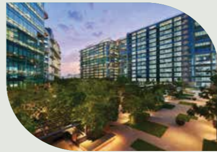
Commerzone Yerwada, Pune
