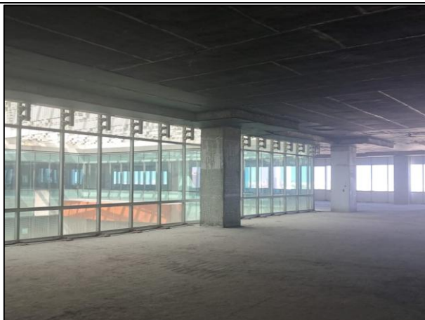
Internal View of the Project
