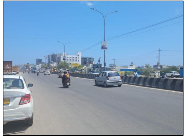
Access road view of the Project
