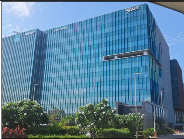
External View of Tower 1A
