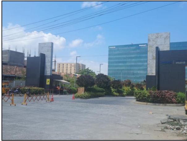
View of the Entry to the Project
