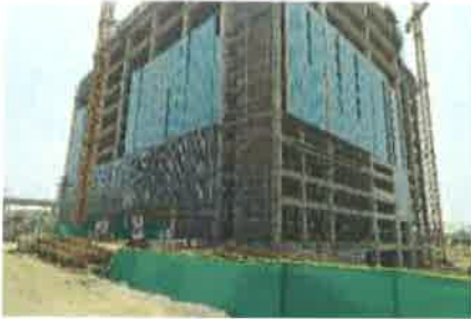
Image 1: External view of Block 1
