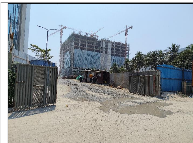
View of the Entry to the Block 1 within the Project
