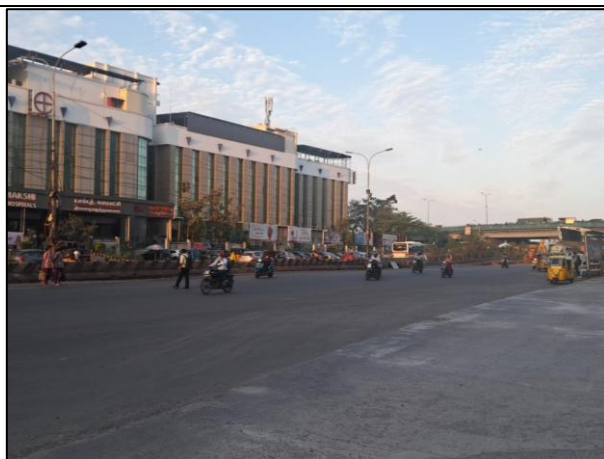
View of the Access Road to the Project
