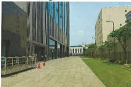
Image 8: External View of Block 3
