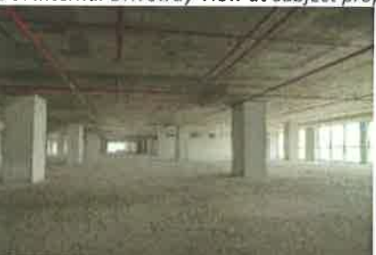
Image 7: Internal view of the property
