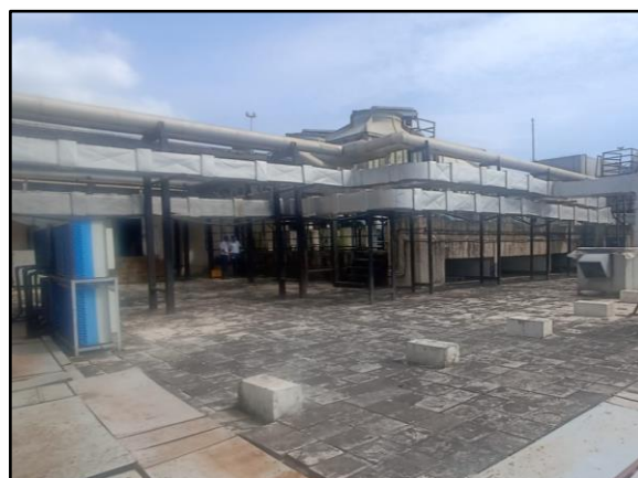
Terrace of Subject Property
