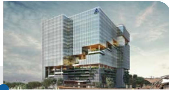
Building 8, Mindspace Madhapur
