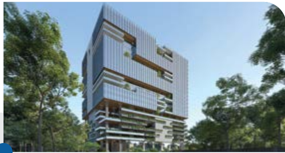
Building 1, Mindspace Madhapur
