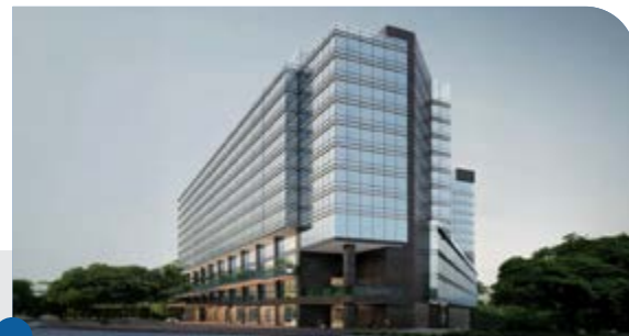
Building 18, Mindspace Madhapur
