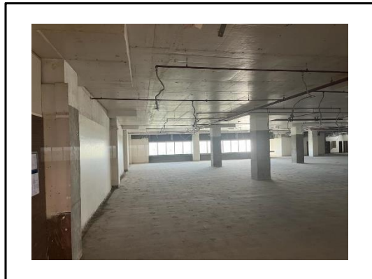
Internal View of Subject Property
