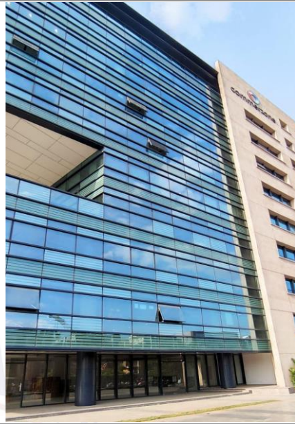
Exterior View of Property
