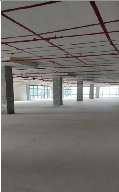
Interior View of Subject Property
