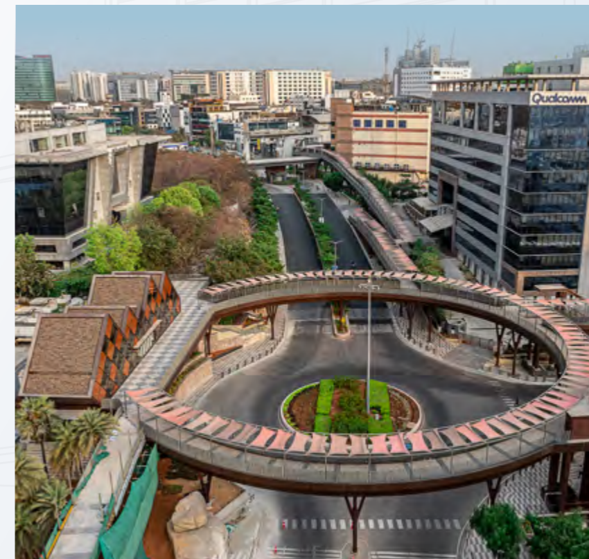
Skywalk: Enhancing connectivity and reducing the carbon footprint
