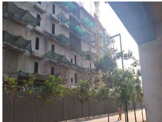
View of Under Construction Building
