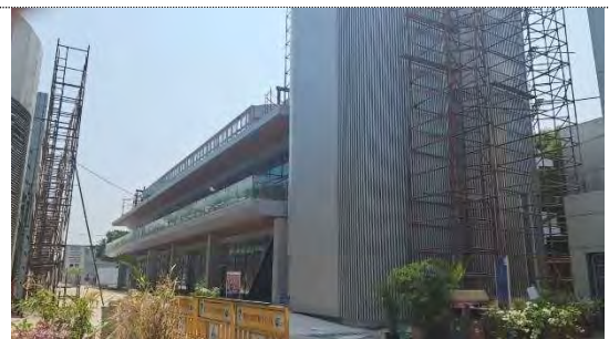
Under Construction – High Street Retail
