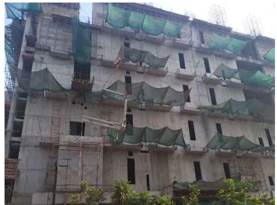
View of Under Construction Building
