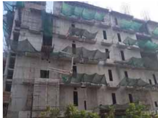
View of Under Construction Building
