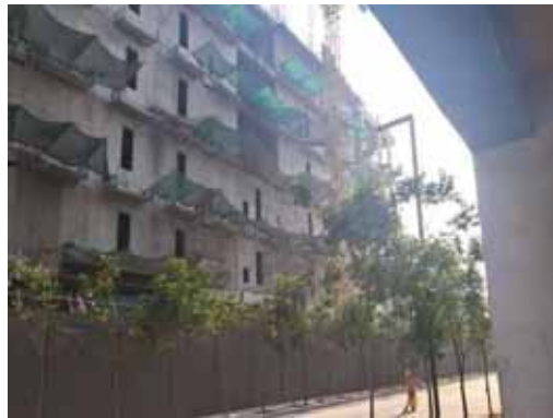
View of Under Construction Building
