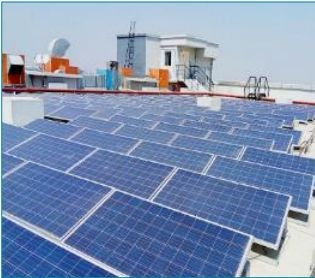
Energy Efficiency - Solar power capacity of 1.8 MW through PV modules on rooftop
